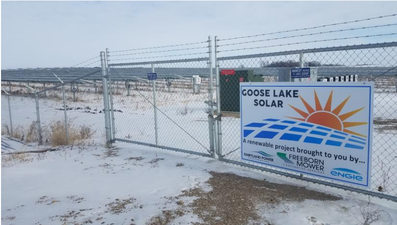
Dairyland Power 1.5 megawatt solar project, Albert Lea, MN
